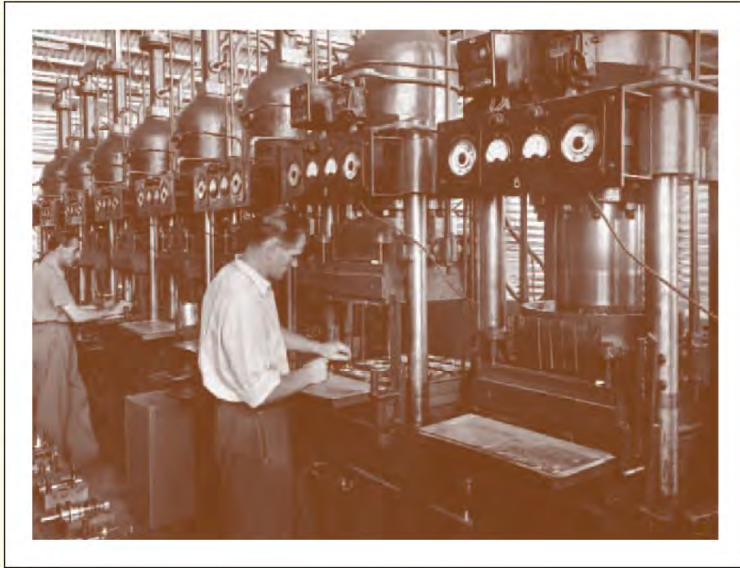
A section of the rubber moulding presses.
